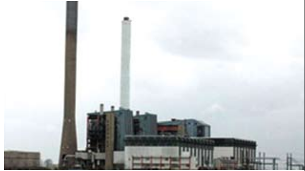
Essent Energie Power Plant
